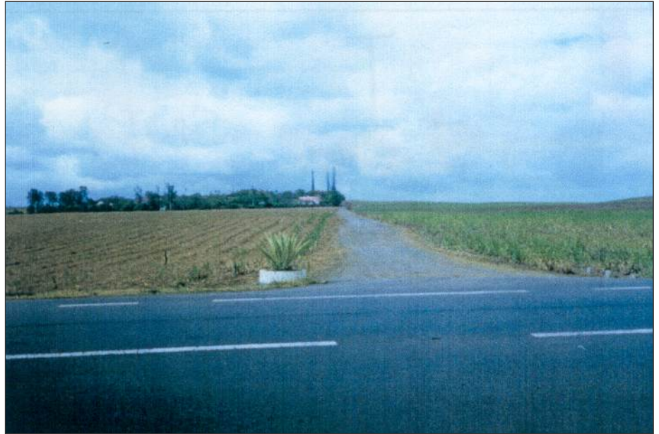
A5 Irrigation Pipeline
